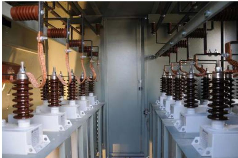
**Fig. 4** Compensating capacitors perform power factor compensation at a utility switching yard.
